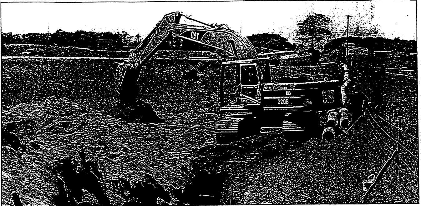
Rothenberger Company's Caterpillar 320B works a yard bucket in placing 16-inch PVC force main along the I-94 right-of-way two miles east of Mattawan.
