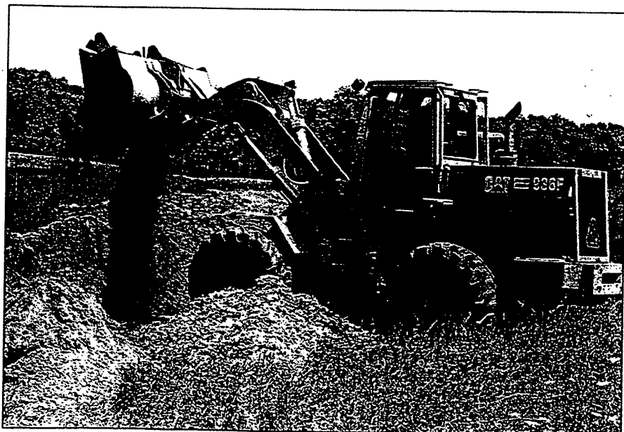
Rothenberger Company's Caterpillar 936F front end loader works a 3-yard bucket to backfill pipe trench along I-94, east of Mattawan.
