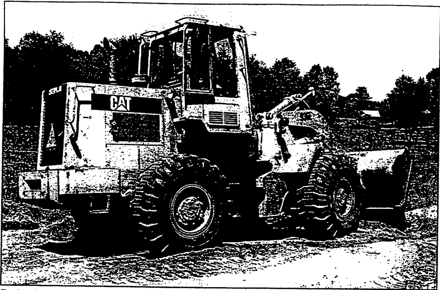
Rothenberger Company uses a Caterpillar 936E loader handling a 3-yard bucket to backfill pipe trench along I-94 right-of-way.
